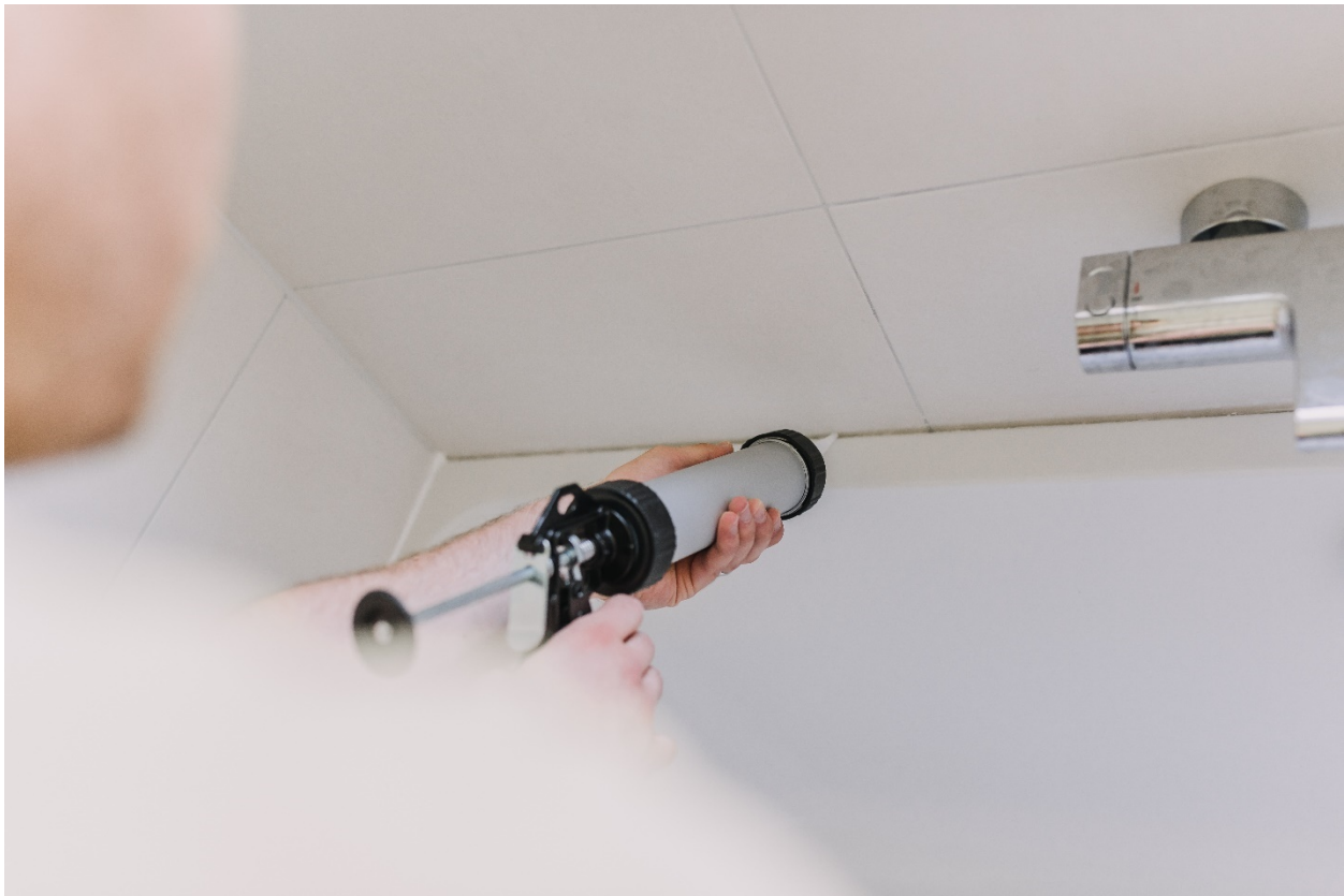
Figure 5. Sealing exterior and interior gaps provides multiple layers of exclusion. Photo: Shutterstock
